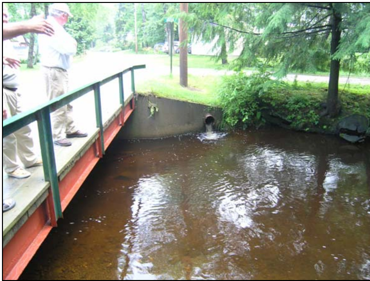
Photo 3: NE wingwall with stormwater pipe.
