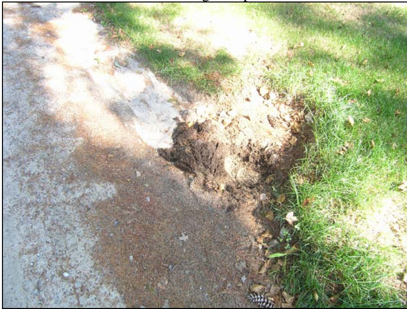
Photo 9: CB3 clogged with pine needles and sediment.
