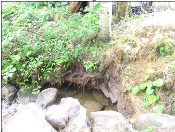
Photo 23: Severe bank erosion at outlet of C19.
