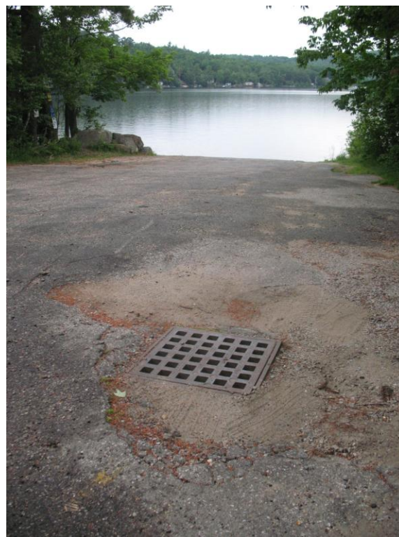
Catch Basin at Boat Ramp (BMP Site 22)
